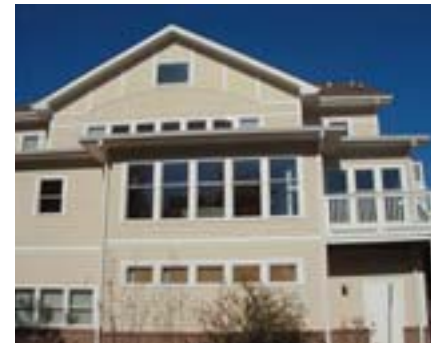
The south side of the Southface office building uses passive solar design. In the winter, the sun shines on the windows and warms the living space, reducing the heating load on the building. In the summer, overhangs shade the windows, reducing the cooling load on the building.
